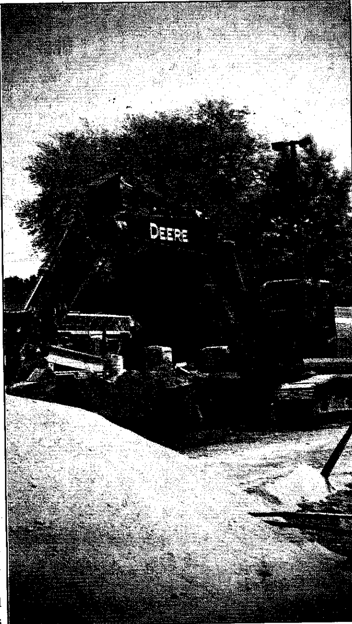
PHOTO BY DREW WOOLERY / PHOTOGRAPHY EDITOR A construction crew does work along South Street across from Grinstead as part of the ESCO project.
